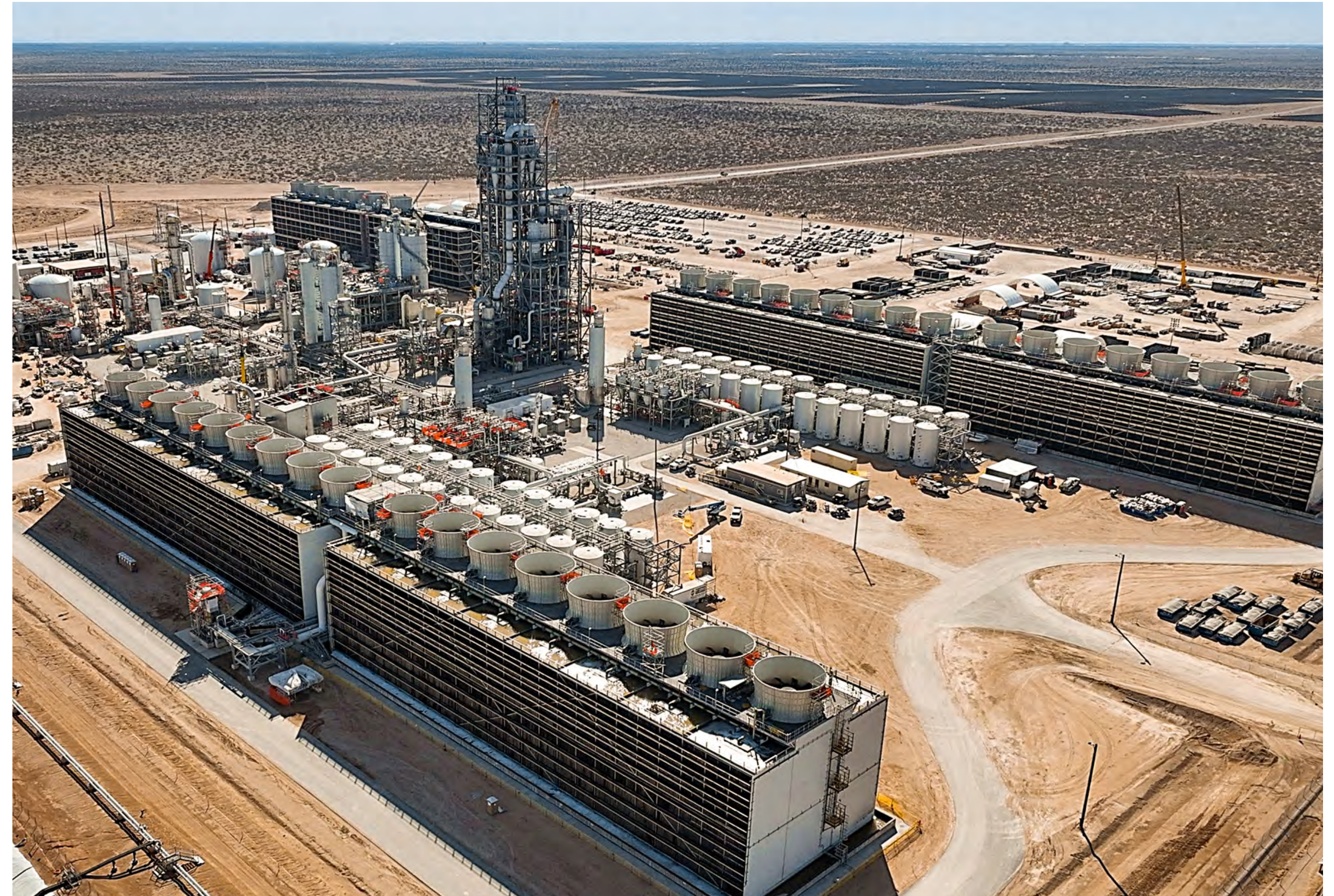
Oxy's STRATOS DAC facility in West Texas
