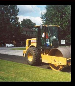
Full-depth reclamation is a process in which the existing surface of deteriorated asphalt roads and the underlying base are pulverized and mixed together to form an upgraded, homogenous new base.
