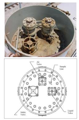
Figure 10: Typical Dome Valve Arrangement
